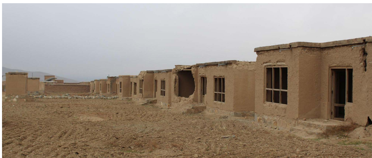
Figure 2. Abandoned dwellings in Barikab settlement (Photo: Samuel Hall 2021)
