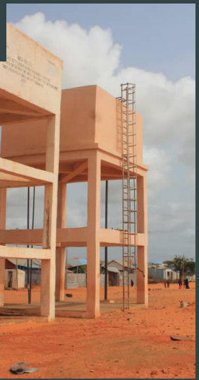
Elevated water tanks in New Kismayo
