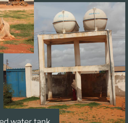
Elevated water tank
