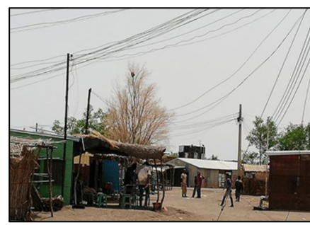
Photo 6 - Electricity available in the market area only
